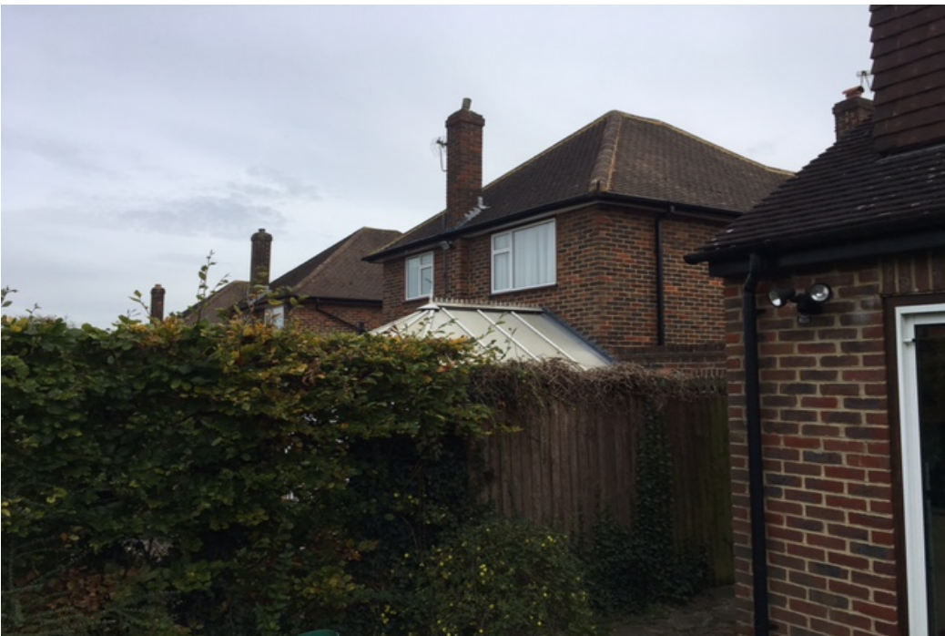
Rear elevation of the neighbouring property no.24 Norman Crescent showing existing 3.5m deep conservatory when viewed from the subject property.
