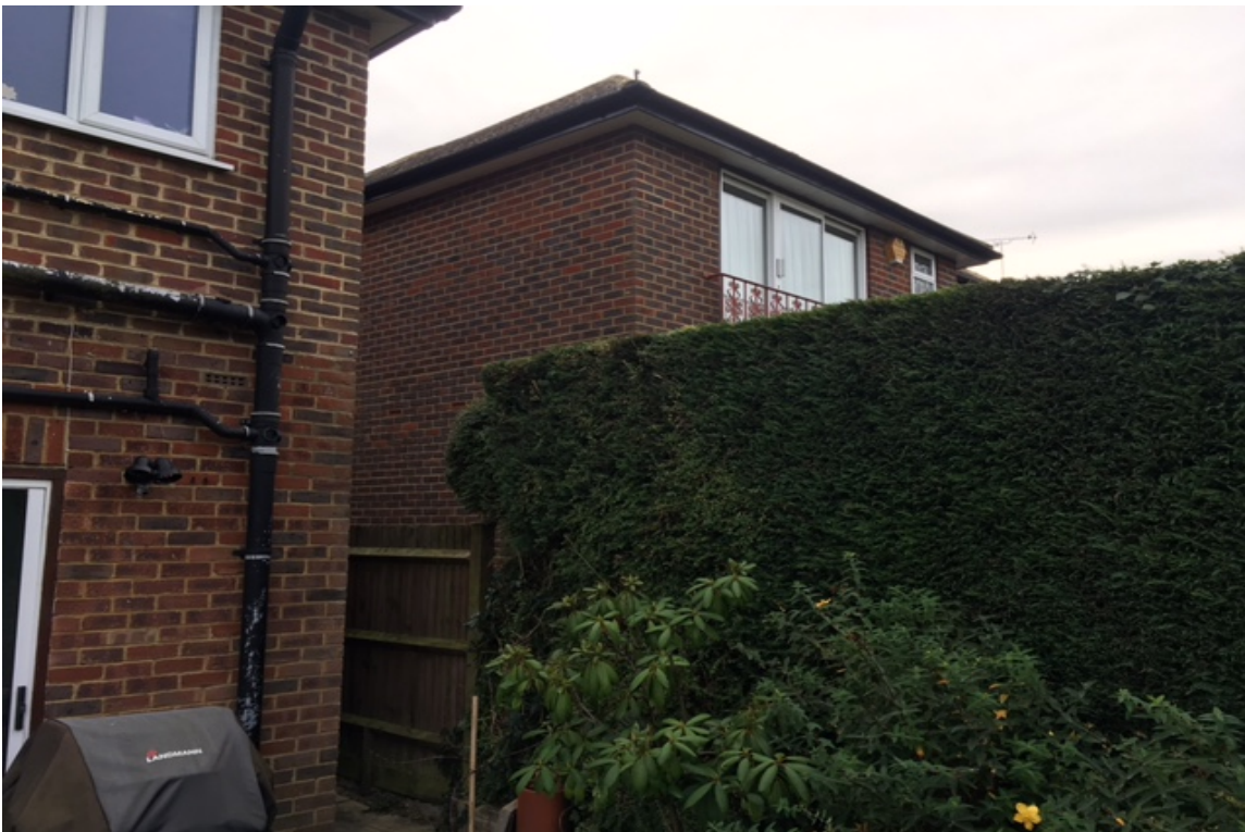
Close up photo showing existing 3.5m high hedge at the common boundary between no.26 and 28 Norman Crescent
