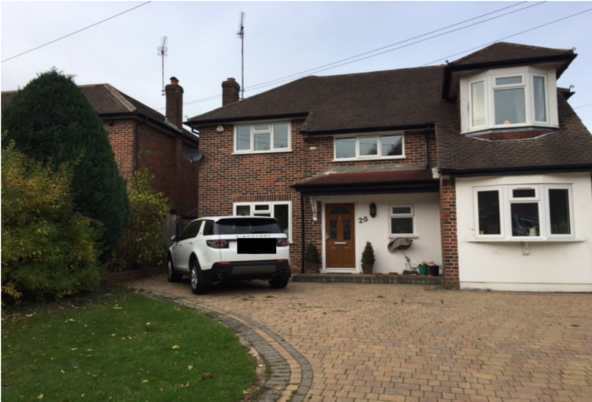
Front elevation of the subject dwelling
