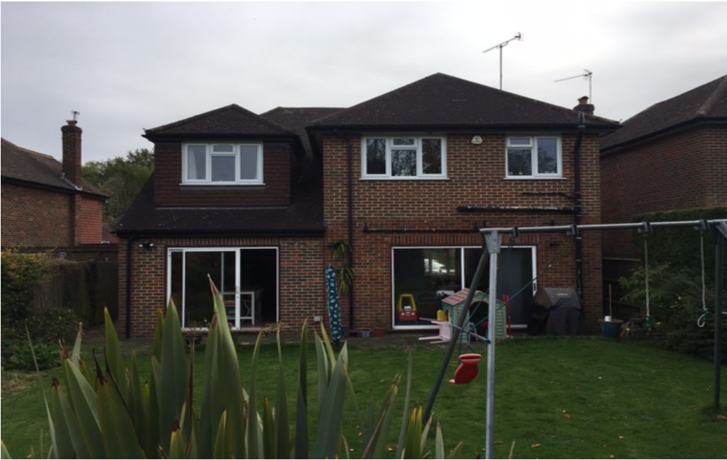
Existing rear elevation of the subject property
