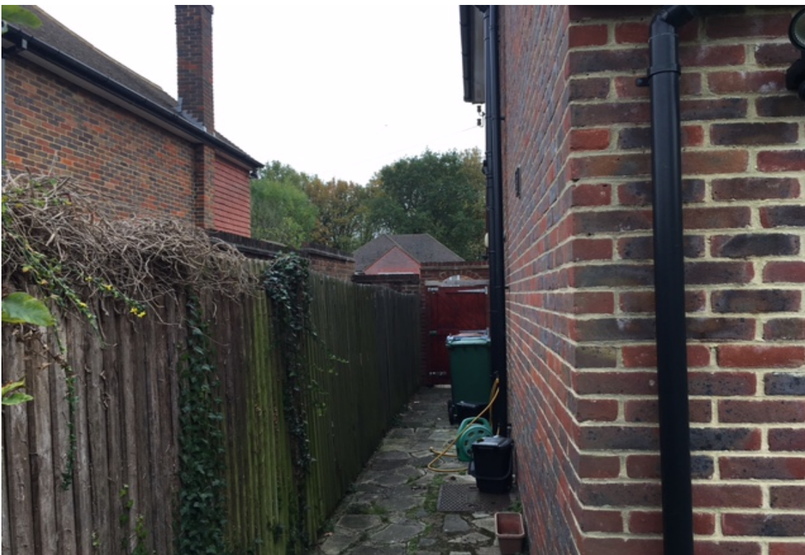
Photograph showing 1.2m separation distance from the existing rear elevation of no.26 and the common boundary shared with no.24
