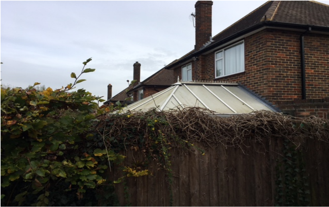
Rear elevation of the neighbouring property no.24 showing the position of the rear conservatory.
